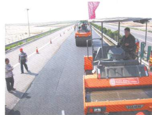
Highway 2.5cm gap-graded wearing layer pavement
